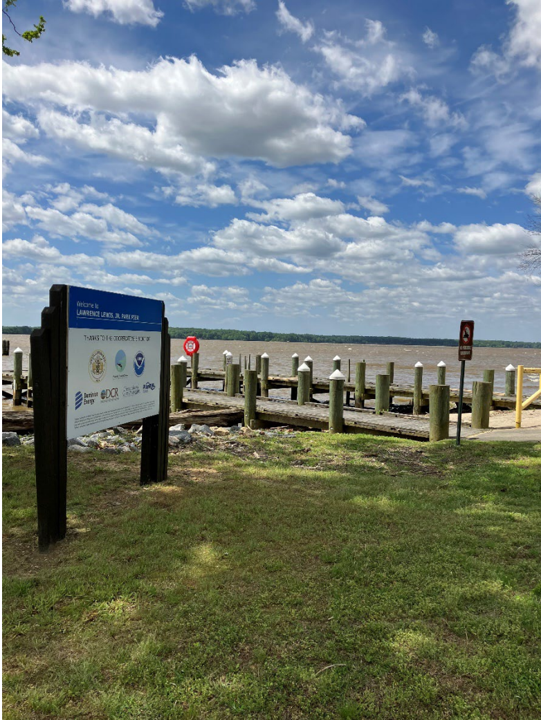
Photo: Lawrence Lewis, Jr., Park Pier, Charles City
