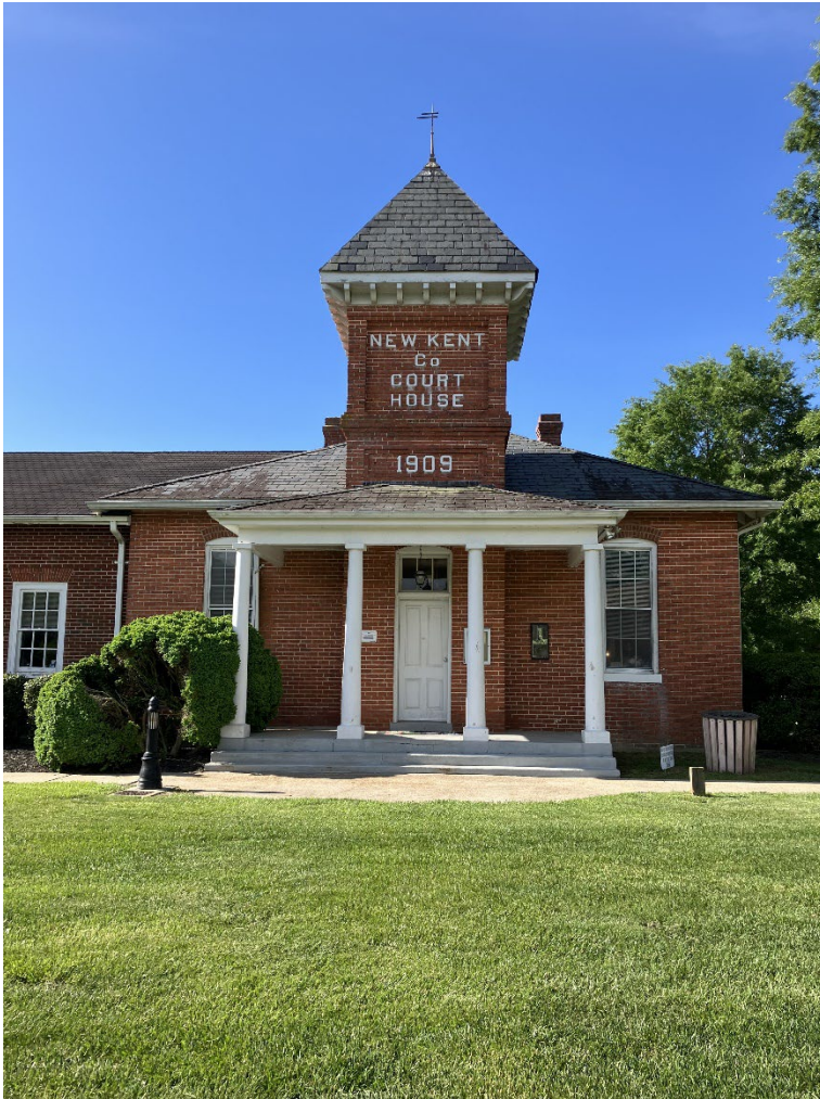
Photo: New Kent County Courthouse
