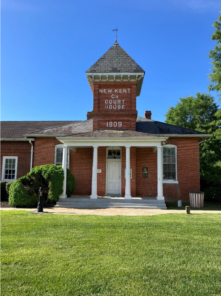
Photo: New Kent County Courthouse
