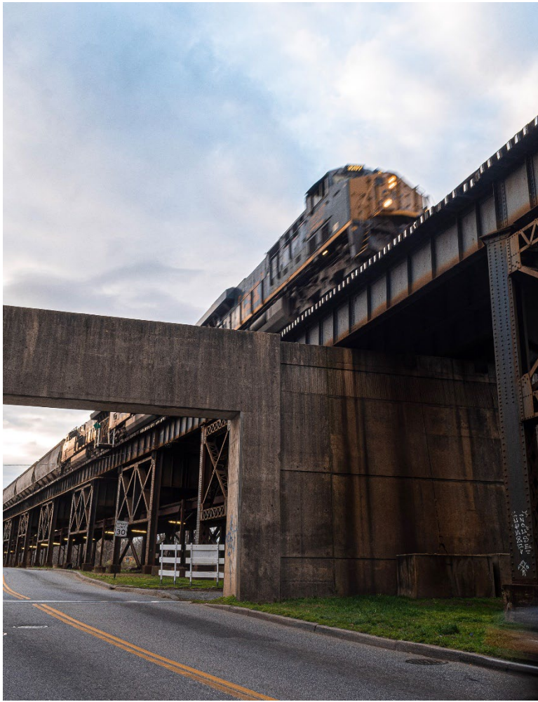
Photo: Train near Canal Walk
