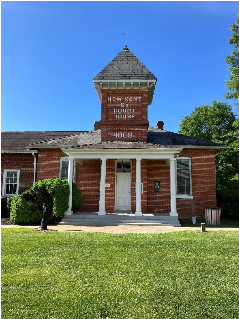
Photo: New Kent County Courthouse
